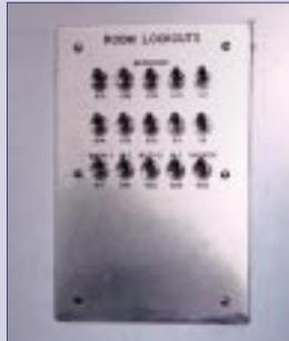
For multiple accommodation, like prison cells and secure hospital rooms, a number of ECO Controllers can be linked to a multi-switch lockout board sited in a supervisor's office, nursing station or prison officers control room. In this way whole areas, floors or particular rooms can be isolated quickly and safely.
